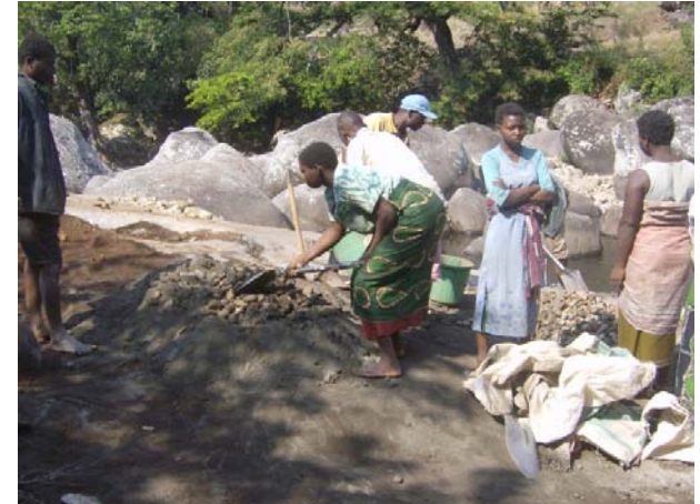
Women preparing cement – participation by the community in Malawi
